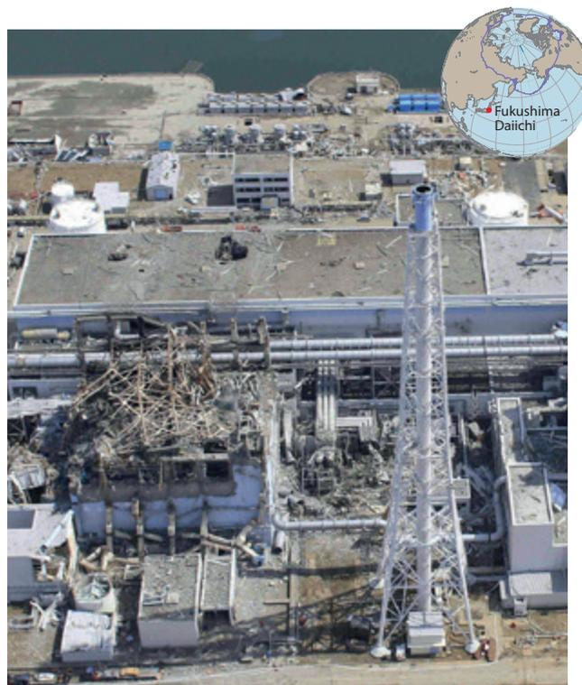
Figure 5.1 Devastation at the Fukushima Daiichi nuclear power plant following meltdown at three on-site nuclear reactor units in March 2011. The inset shows the location of the Fukushima Daiichi NPP.
